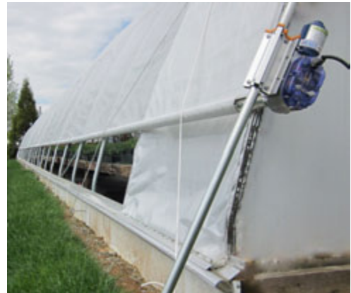
FIGURE 1 MOTORIZED ROLLUP SIDEWALL CURTAIN
