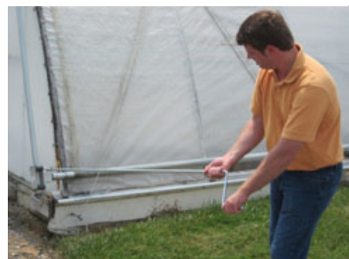
FIGURE 3 MANUAL ROLLUP CURTAIN DRIVE SYSTEM
